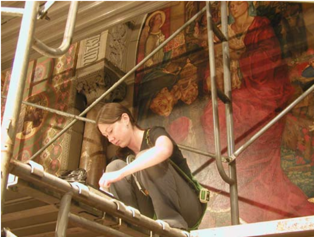
Denyl Cloughly, an art conservator with Griswold Conservation in Los Angeles, mixes paints to be used on the mural over the altar in the Chapel. Ms. Cloughly worked with Darren Martin, Timothy Rudolph and Robert O'Connell of O'Connell International Arts for two weeks in June as they removed soot from the murals, columns and stained glass windows. The soot was a result from a small fire in December. During the cleaning period, services usually held in the Chapel were moved to the church.
